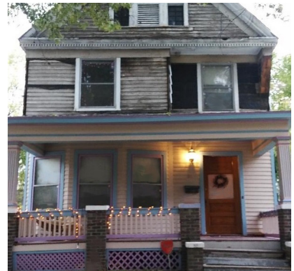
PROJECT EXAMPLE: BEFORE
