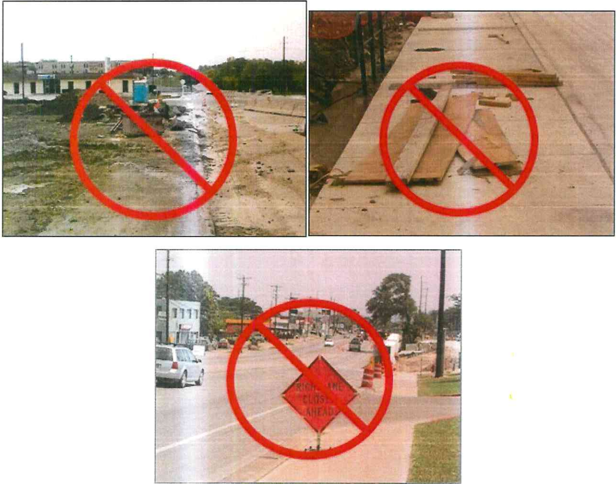
Figure 8. Pedestrian sidewalks and paths that are left open for use must be kept clear (source: TTI)
