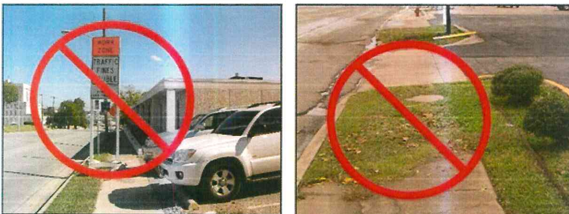
Figure 19. The pedestrian detour route should be continuous and free of obstacles (Source: TTI)
