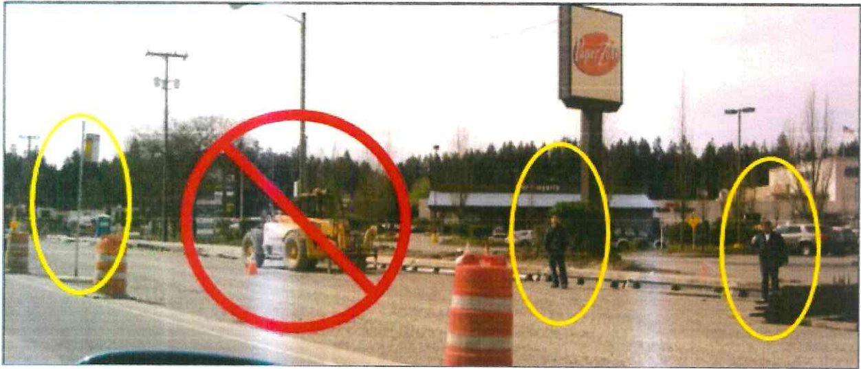
Figure 7. Transit users should not be forced to walk through active work spaces to reach transit stops (Source: TTI)
