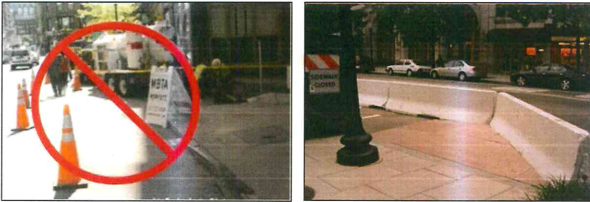
Figure 15. Proper separation devices must be used when diverting pedestrians into travel, parking, or bicycle lanes (Source: J. Barlow, Accessible Design for the Blind ; TTI)
