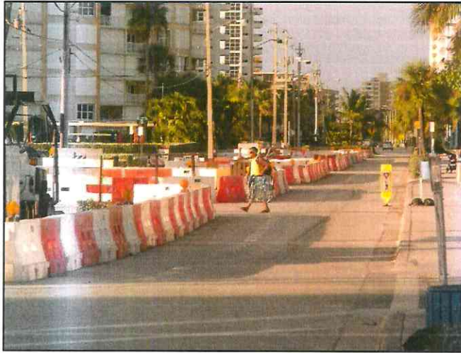
Figure 5. Example of longitudinal channelizers used to separate pedestrians from work spaces (source: TTI)
