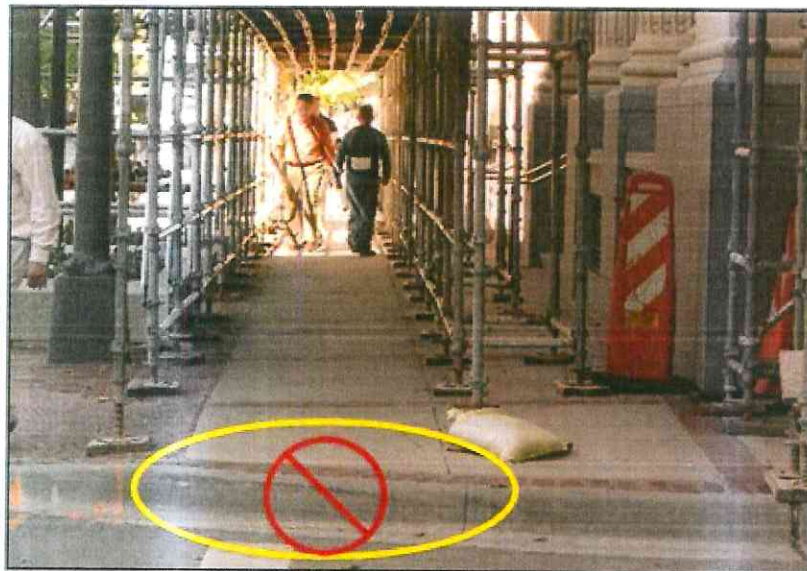
Figure 13. Proper temporary curb ramps are required wherever the diversion path traverses a curb (Source: TTI)
